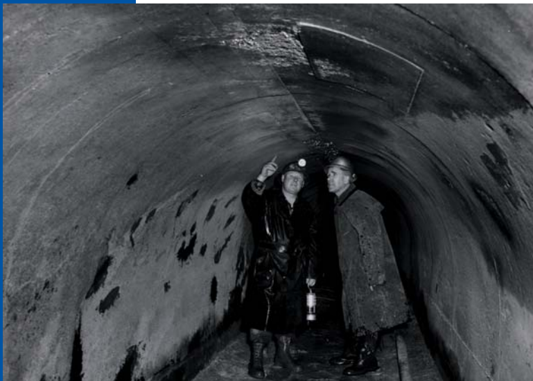
Installation of Sturgeon Point treatment plant transmission main, 1960
