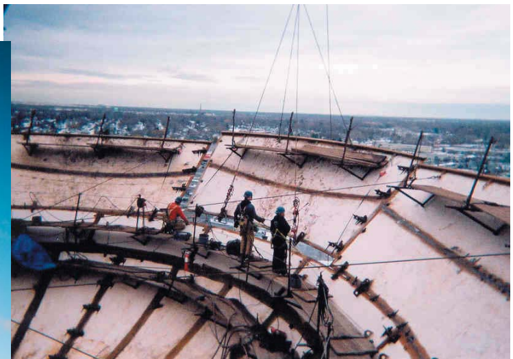
Workers erect the bowl on the Colvin Boulevard storage tank in Tonawanda, 2003
