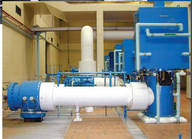
Above: Dedication of Guenther pump station, 1972. Right: Vertical turbine pumps at Van de Water treatment plant, 2003
