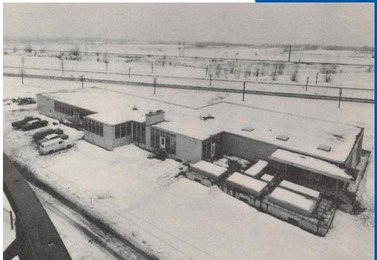
Operations Control and Service Center, 1957
