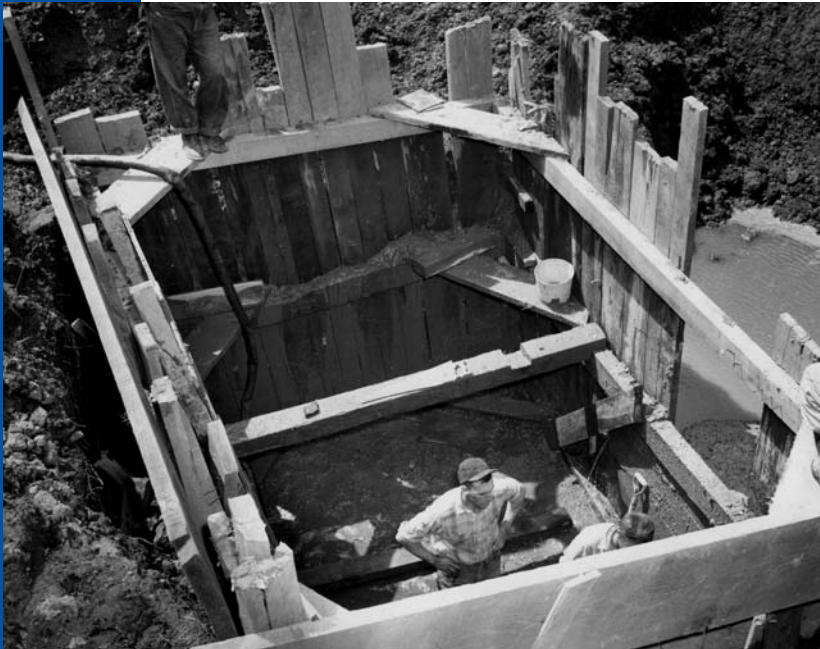
Harlem Road pump station construction , 1956
